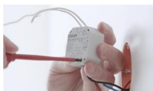
**01** Connect the DALI ACU BT to the mains and DALI wires.
